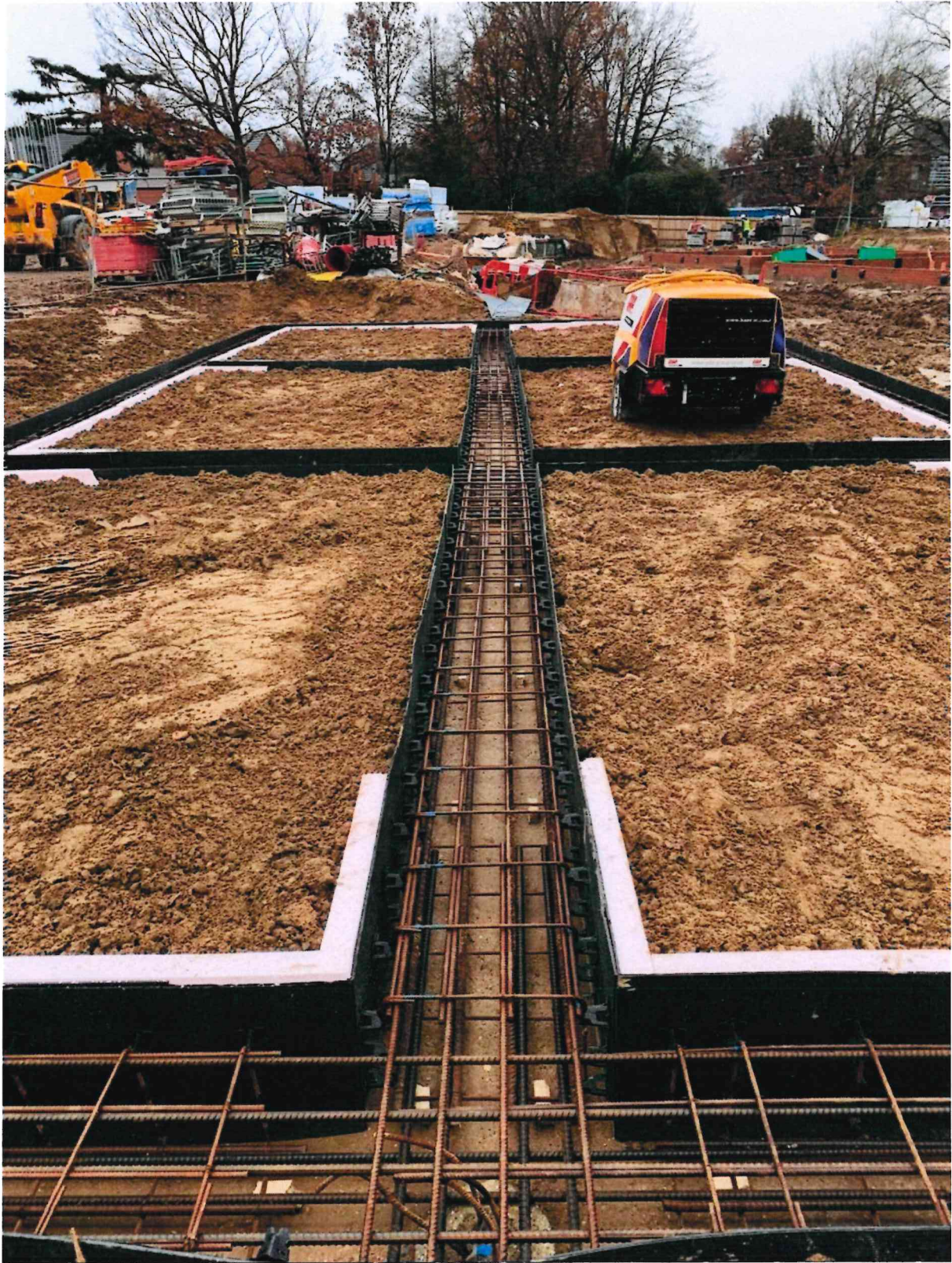
Well Presented Ground Beams
