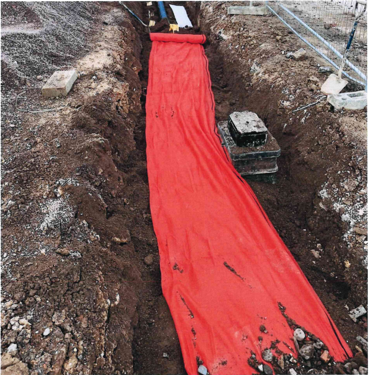
Orange Debris netting placed over services.
