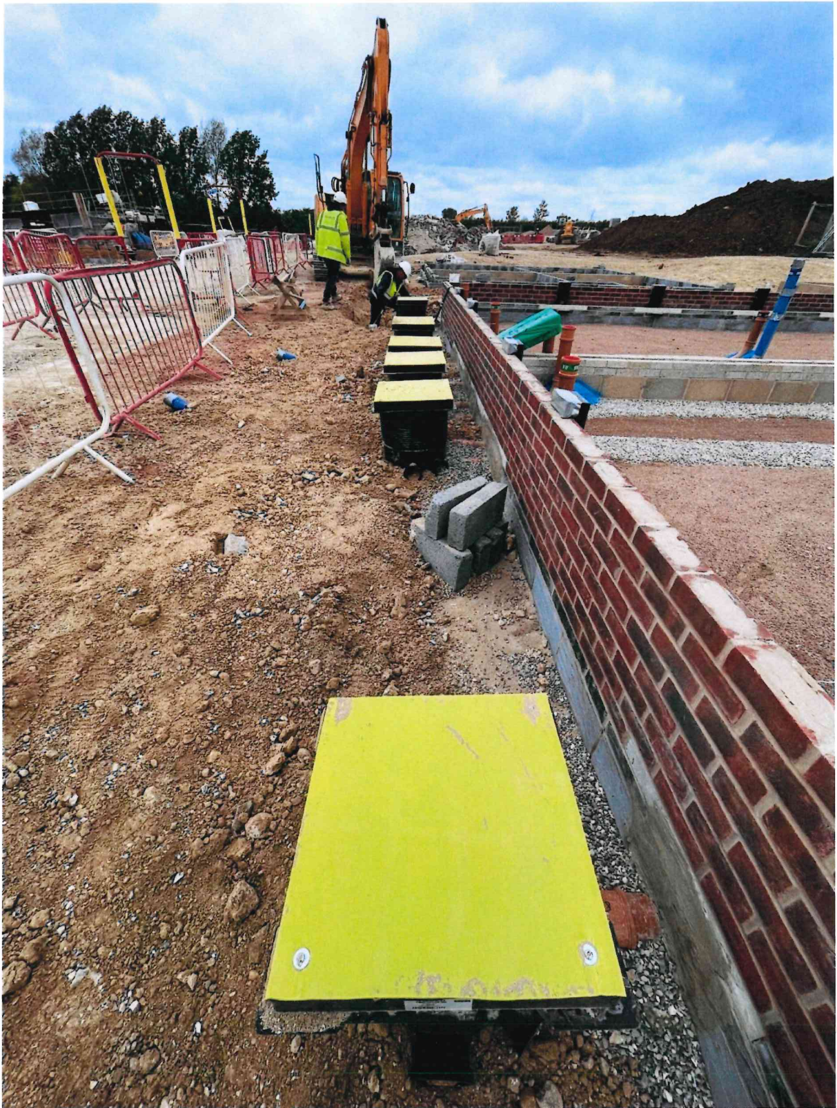
Manhole Protection in place
