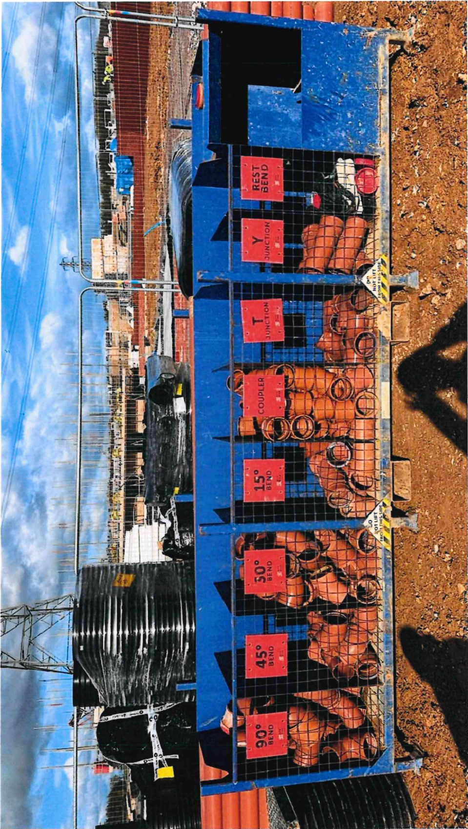
Site stack being utilised for drainage fittings
