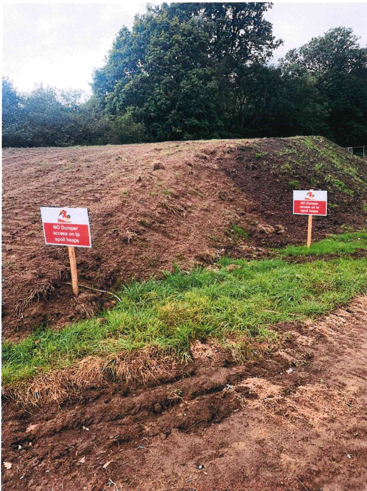
Clear signage stating NO DUMPER ACCESS ON SPOIL HEAPS
