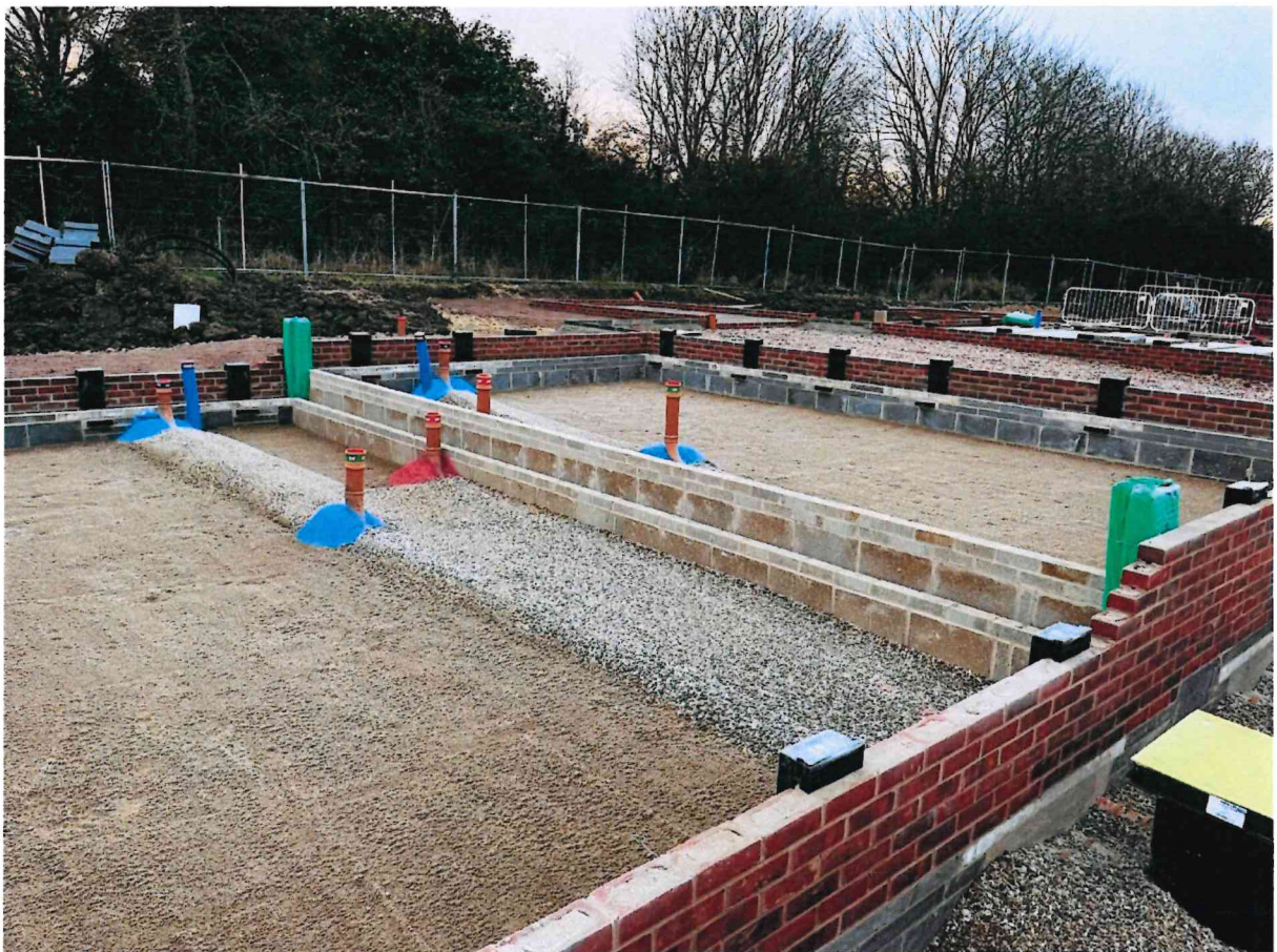
Well Presented Oversite/Internal Drainage
