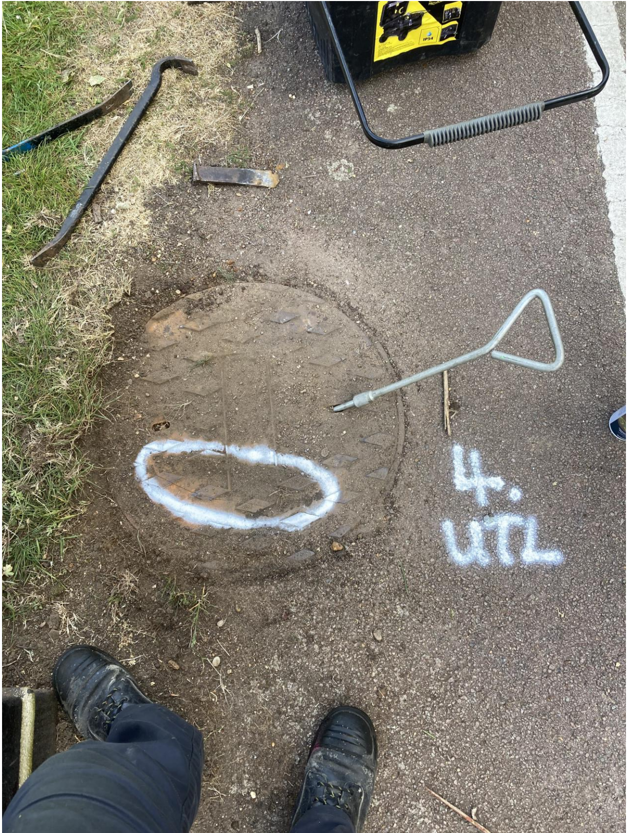
Fig 1: MH not lifted due to seized frame and cracked/damaged cover.
