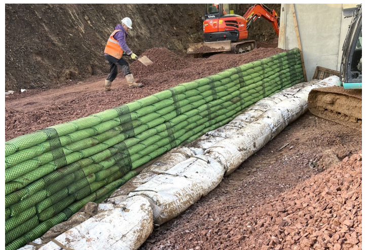
Fig 12. Geogrid wrap-around.
