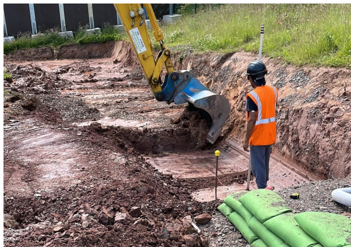
Fig 2. Excavating multiple steps.
