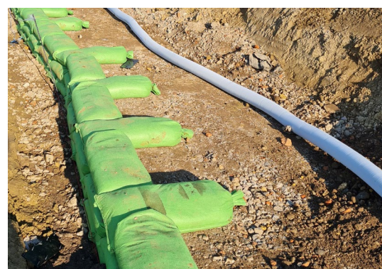
Fig 9. Laying drainage pipe.
