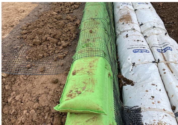
Fig 13. Geogrid wrap-around placement.
