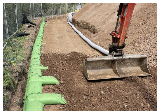
Fig 8. Placing the backfill material.
