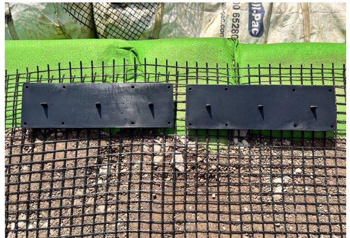
Fig 11. Interlocking plate placement.
