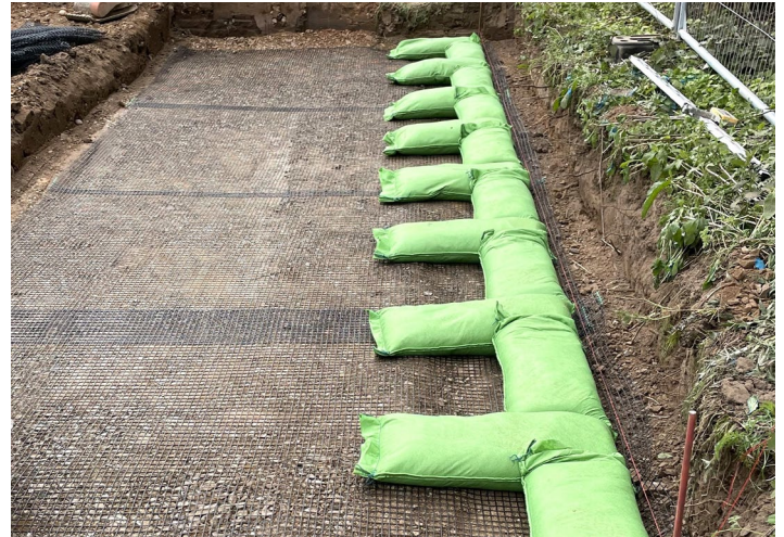
Fig 10. Geogrid placement.
