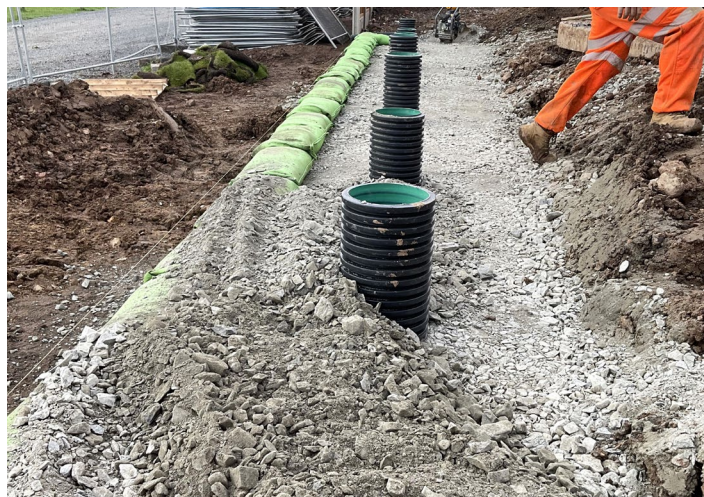
Fig 14. Placement and backfilling of post sleeves.
