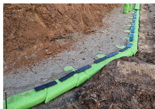
Fig 7. Laying first row of bags and second row of interlocking plates.
