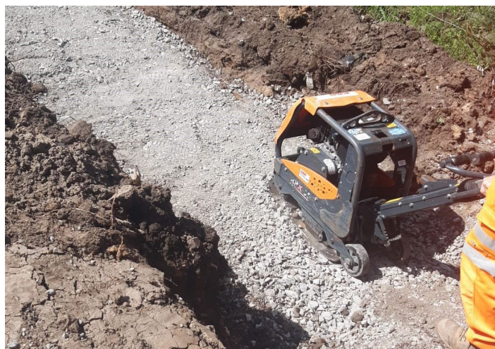
Fig 3. Compacting the foundation.
