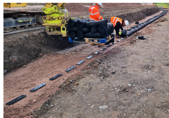
Fig 6. Laying the first row of interlocking plates.
