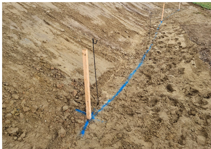
Fig 1. Setting out the toe of wall.
